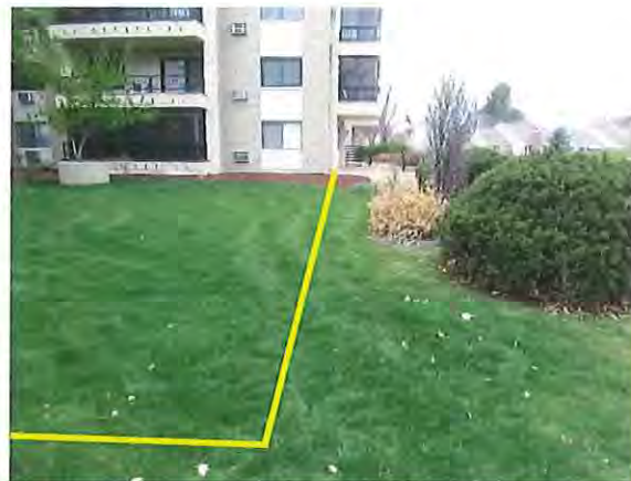
Figure 1. Overall view of landscaped area at north corner of Building 244. Yellow lines denote approximate extent of foundation wall and parking garage, below.
