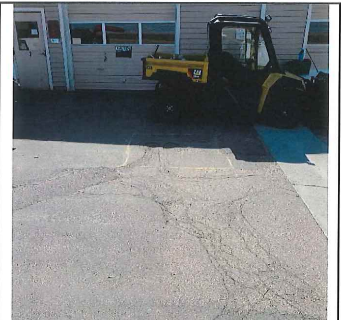
Asphalt Repairs - 5' x 5'
