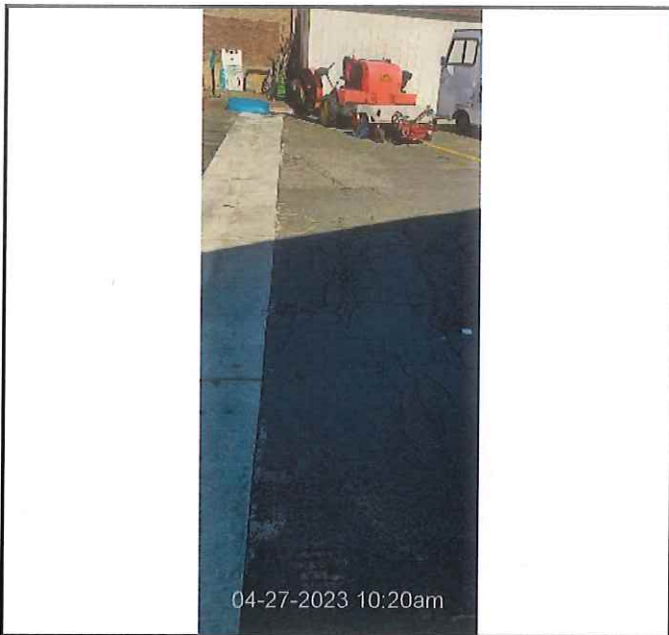
Asphalt Repairs - 4' x 14'
