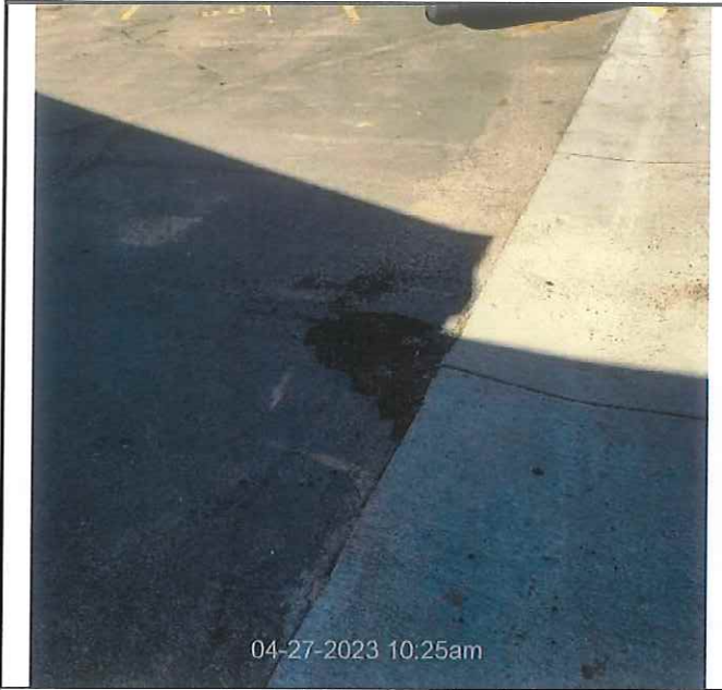
Asphalt Repairs - 9' x 4'
