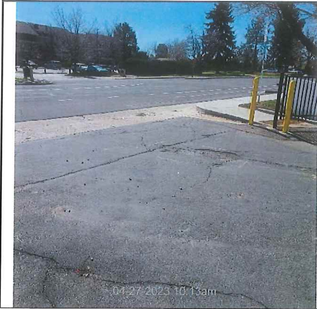
Asphalt Repairs - 22' x 15'
