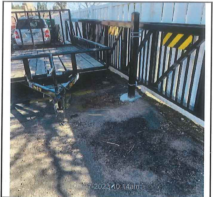
Asphalt Repairs - 4' x 5'
