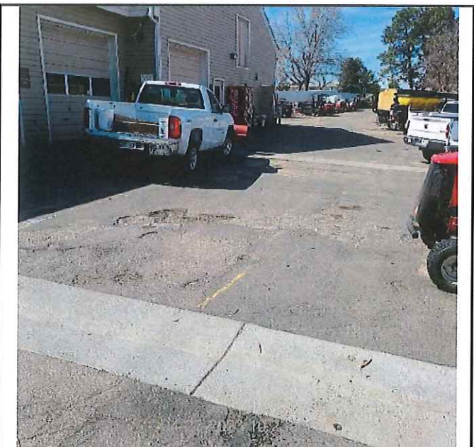
Asphalt Repairs - 32' x 32' Picture #1
