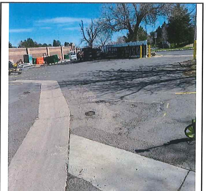
Asphalt Repairs - 184 SF or 10' x 10' and 6' x 14'
