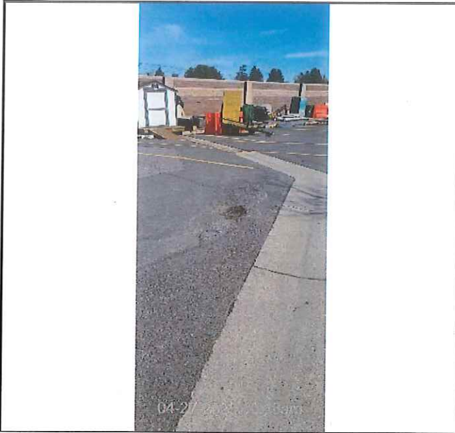
Asphalt Repairs - 4' x 12'
