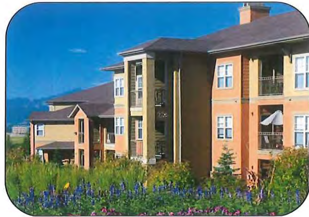
Talon Hill Apartments Colorado Springs, CO Full Exterior Repaint
