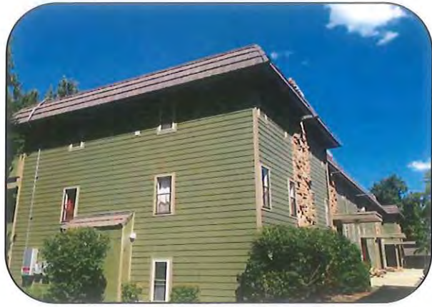
Remington Post HOA Boulder, CO Full Exterior Siding Replacement & Paint
