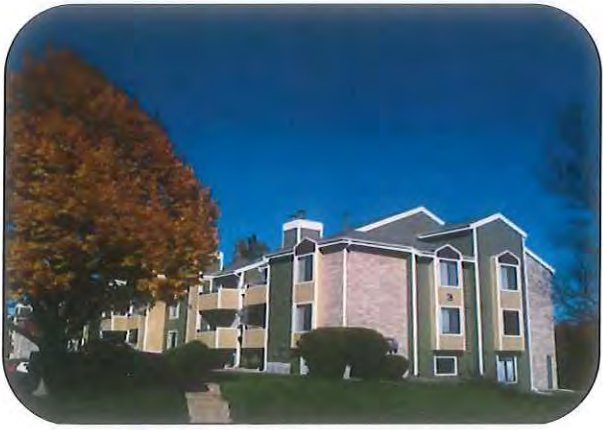
Hunters Ridge Apartments Denver, CO Full Exterior Siding Replacement and Paint
