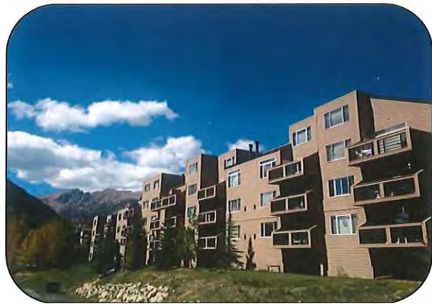
Watch Hill Condominiums Silverthorne, CO Full Exterior Repaint
