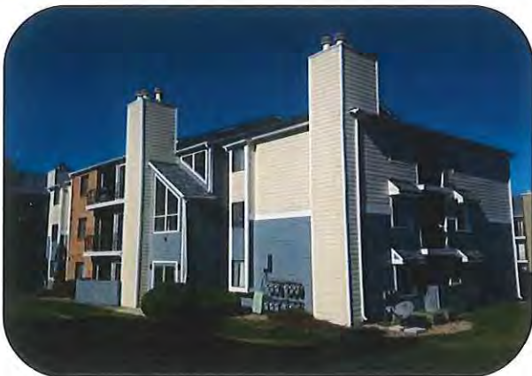
Sunchase Apartments Aurora, CO Full Exterior Siding Replacement & Paint
