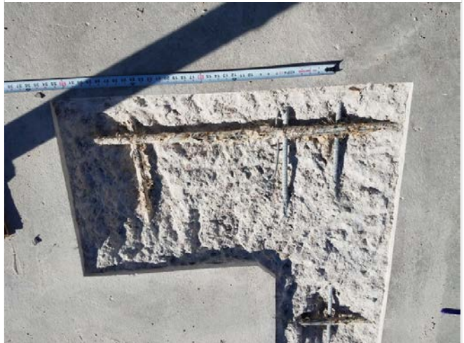
Photo 4 – Typical PT tendon bundle.
