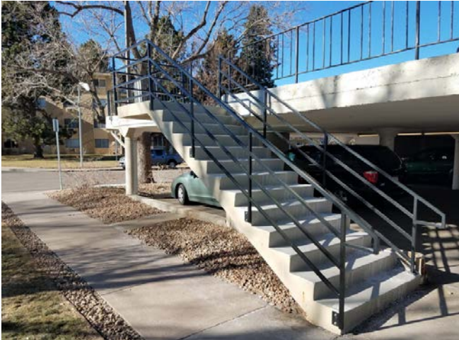
Photo 5 – Typical stair layout and railings.
