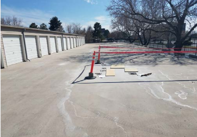
Photo 1 – Exploratory openings of tendons running in the east-west direction.
