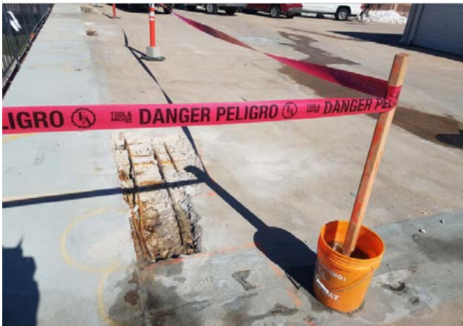
Photo 3 – Failed PT tendons at the anchors due to corrosion.
