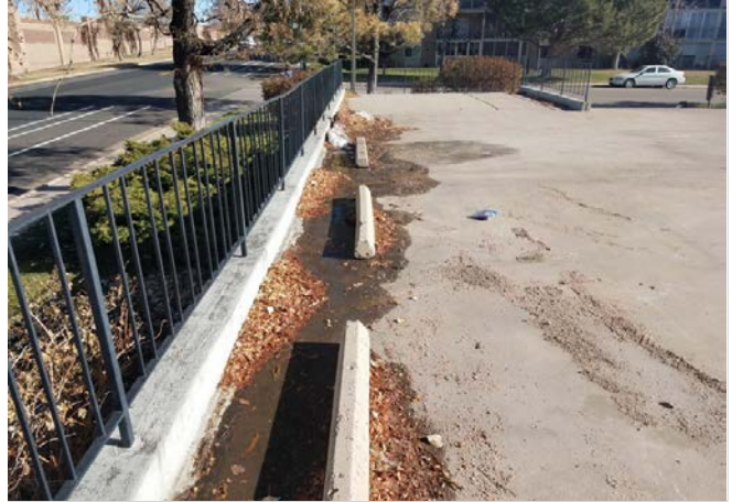
Photo 2 – Perimeter railing at Structure #2. Typical of perimeter railings at all structures.
