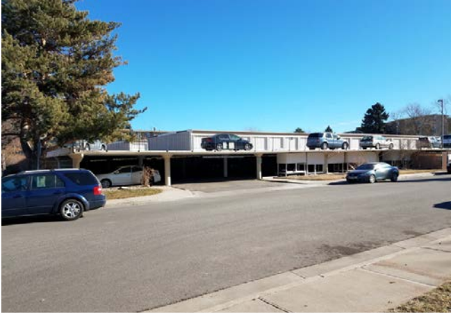
Photo 1 – View of Structure #2 viewed from the west. Typical single supported level construction.
