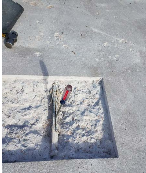
Photo 2 – PT tendon penetration test. (Used to determine if tendon is stressed)
