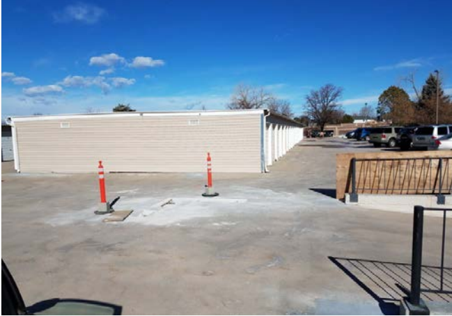
Photo 1 – South end of Structure 2 at typical exploratory openings at PT tendons.
