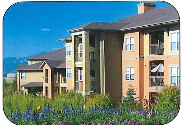
Talon Hill Apartments Colorado Springs, CO Full Exterior Repaint
