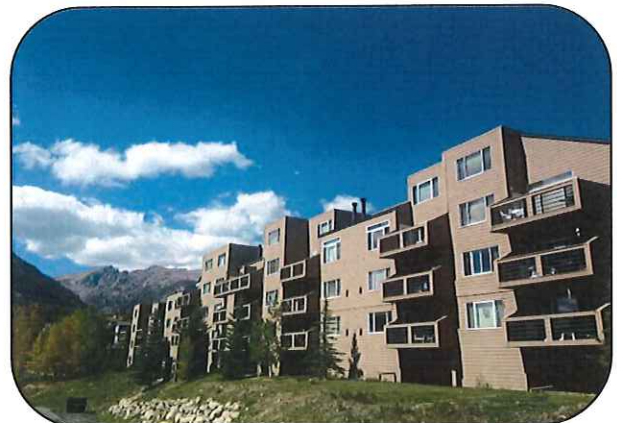
Watch Hill Condominiums Silverthorne, CO Full Exterior Repaint
