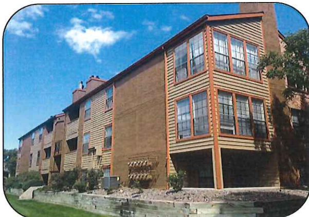
Winridge Apartments Aurora, CO Siding Replacement/ Full Exterior Repaint
