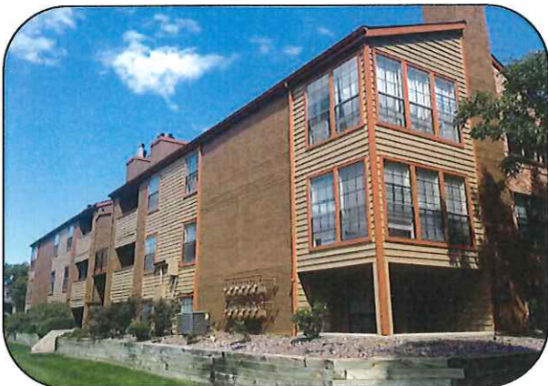
Winridge Apartments Aurora, CO Siding Replacement/ Full Exterior Repair
