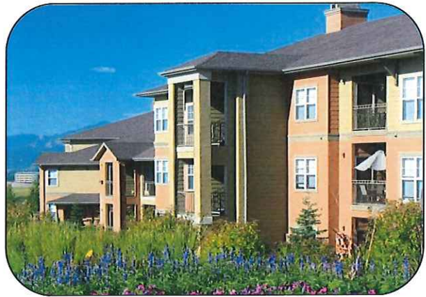
Talon Hill Apartments Colorado Springs, CO Full Exterior Repair
