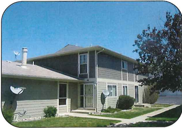
Raintree HOA Denver, CO Full Exterior Siding Replacement & Paint
