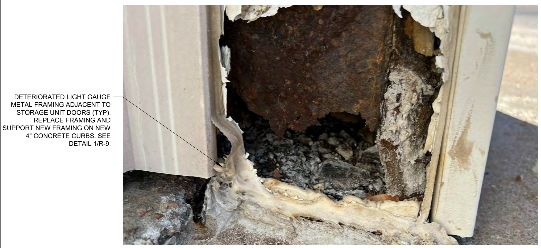
DETERIORATED FRAMING AT STORAGE UNITS NOT TO SCALE
