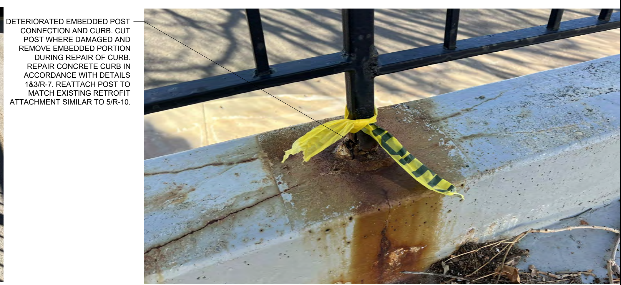
DETERIORATED EMBEDDED RAILING POST NOT TO SCALE
