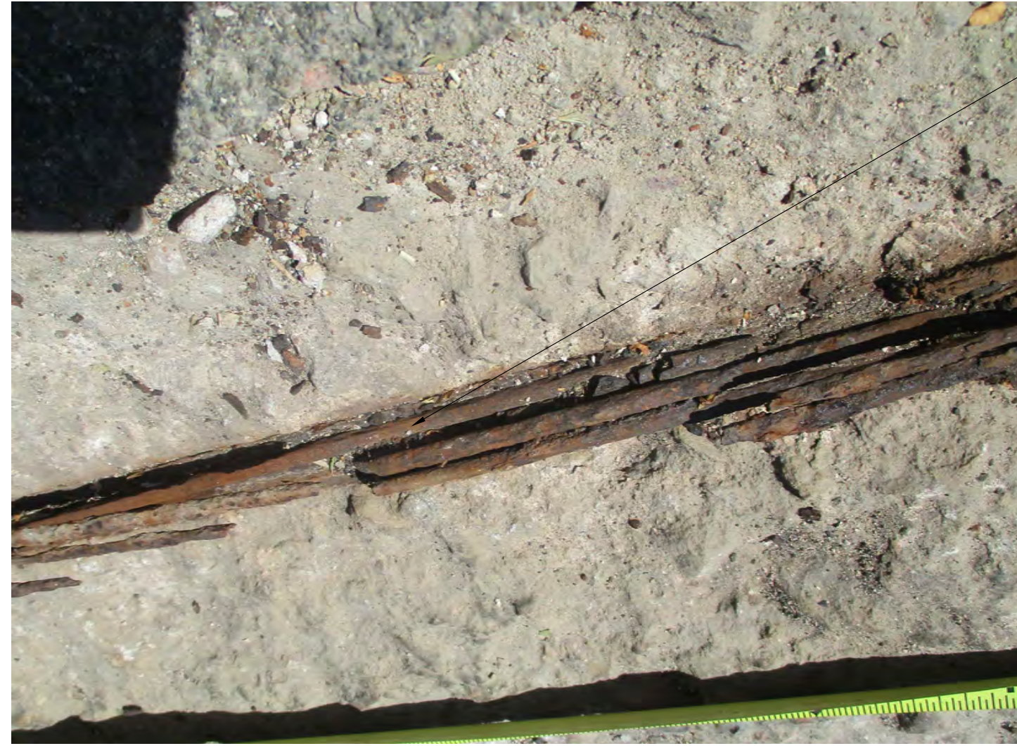
TYPICAL BROKEN TENDON. SEE 2/R-4 AND 1/R-5 FOR REPAIR DETAILS.
